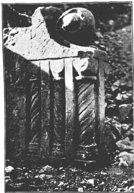
NORMAN BENCH END DORMITORY UNDERCROFT.
